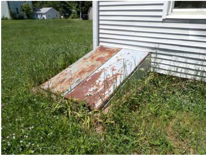
Typical bulkhead deterioration
