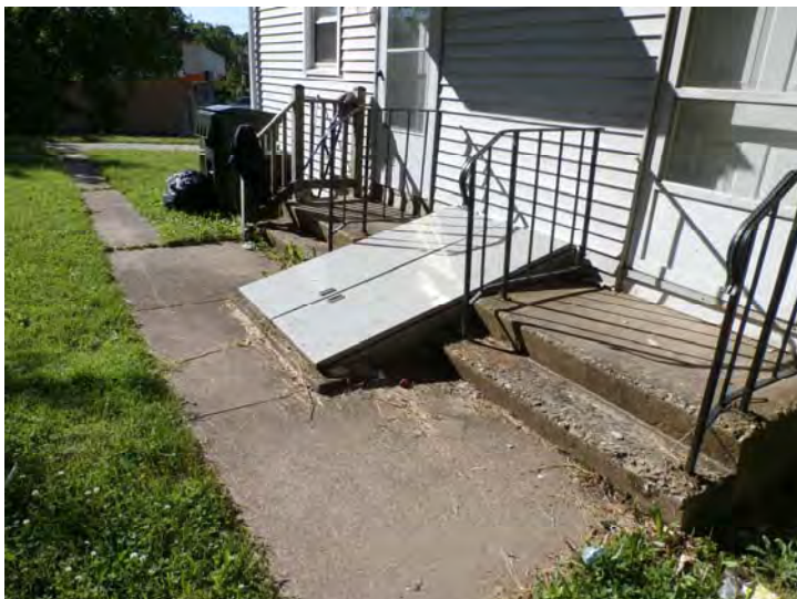
Typical example of concrete age related deterioration
